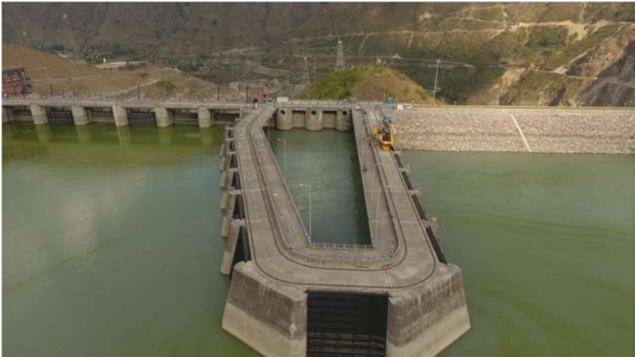
Fig. 6(c) : Pictorial View of Kol Dam Decanting Chamber in Operation
