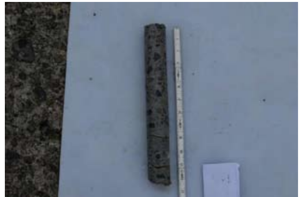
Fig. 12 : Concrete core from “Red area”
