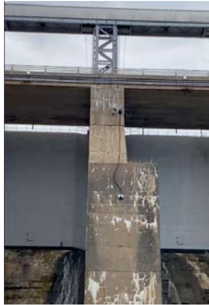
Fig. 4 : Acoustic data collection on a spillway pier
