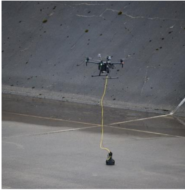
Fig. 5 : Acoustic data collection on a spillway slab
