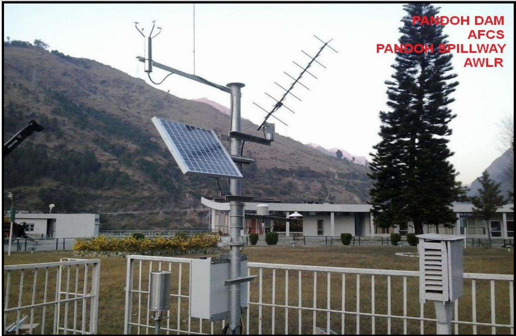
Full Climatic Station Installed at Pandoh Dam, Elevation 2949 ft
