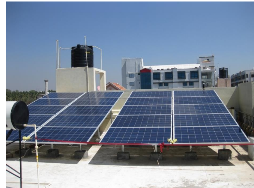
Residential house at kengari– 5 kW
