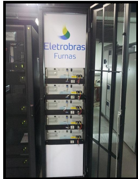
Figures 4 and 5: Tests on lithium-ion batteries in the factory and final installation in the company (Photos: Alexandre Pinhel)
