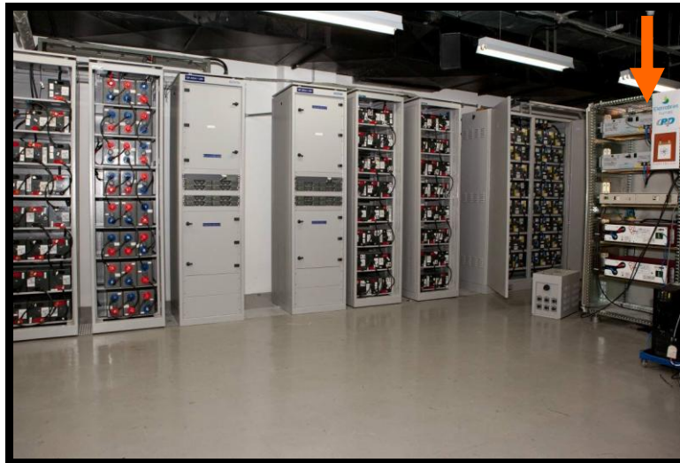
Figure 1: Comparative Overview: Backup systems with VRLA batteries and lithium-ion Experiment indicated by the red arrow on the far right (Photo: Alexandre Pinhel)
