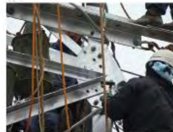
Figure 8 Remove gusset plate
