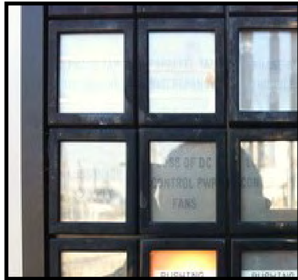
Figure 7 warning signal of Bushing On-Line Monitoring System at Annunciator
