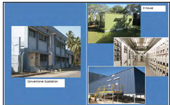
Fig 5-Conventional DSS Vs E House DSS
