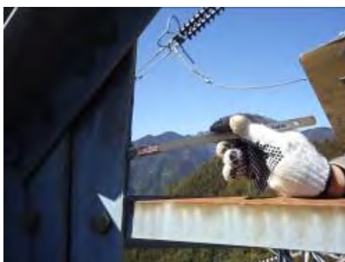
Figure 24 Applying metallic putty
