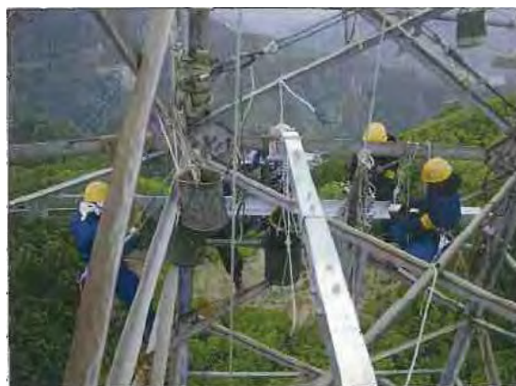
Figure 12 Defective plate replacement with jig
