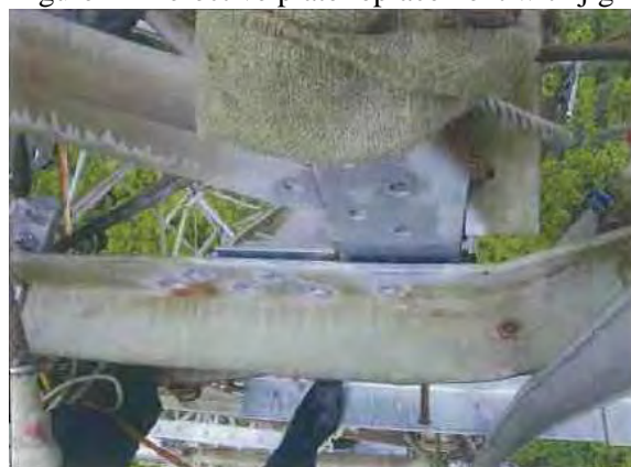
Figure 14 After removing the defective gusset-plate
