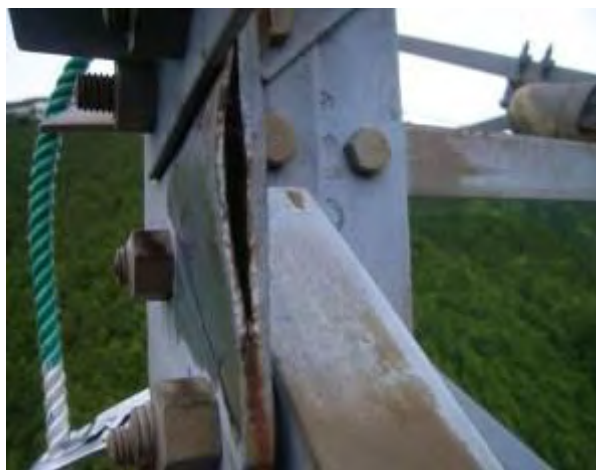
Figure 1 Lamination example (Gusset-plate connecting the cross arm and steel tower body for 275 kV transmission line)
