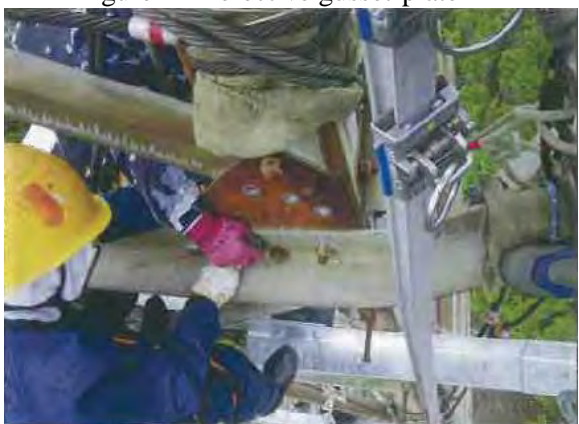
Figure 13 Removing the defective gusset-plate
