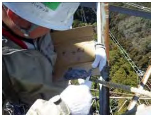
Figure 23 Preparation of metallic putty
