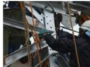
Figure 9 Remove gusset plate
