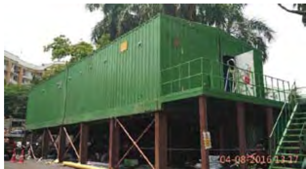
Fig-6-E house in its final stages of implementation at a Tata Power Substation
