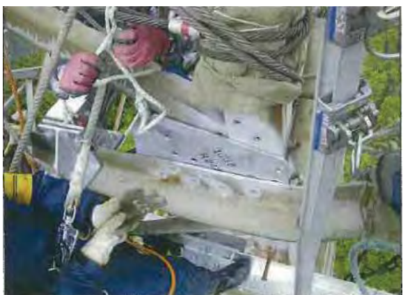
Figure 15 Inserting a new gusset-plate
