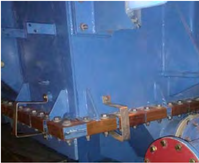
Fig. 14 Actual view of copper strip at tank bell joint
