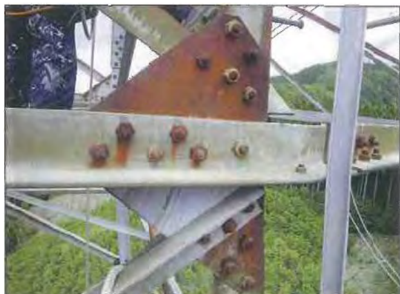
Figure 11 Defective gusset-plate
