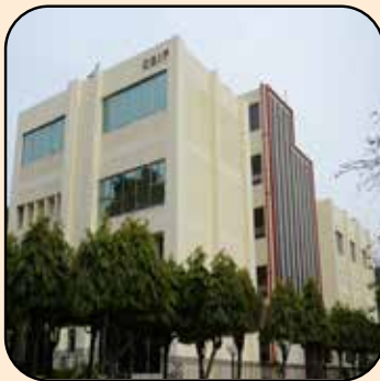
CBIP office at Chanakyapuri, New Delhi (1980 onwards)
