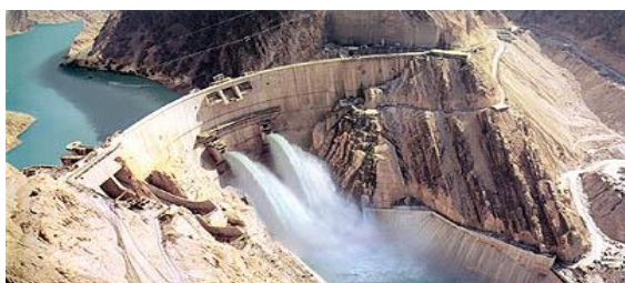
Figure 1: View of Karun 3 Dam and Power Plant
