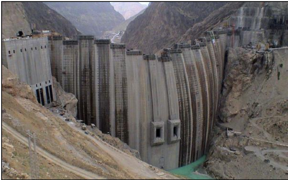
Figure 1. Construction progress at the start of Karun 4 reservoir impounding (March 25, 2010)
