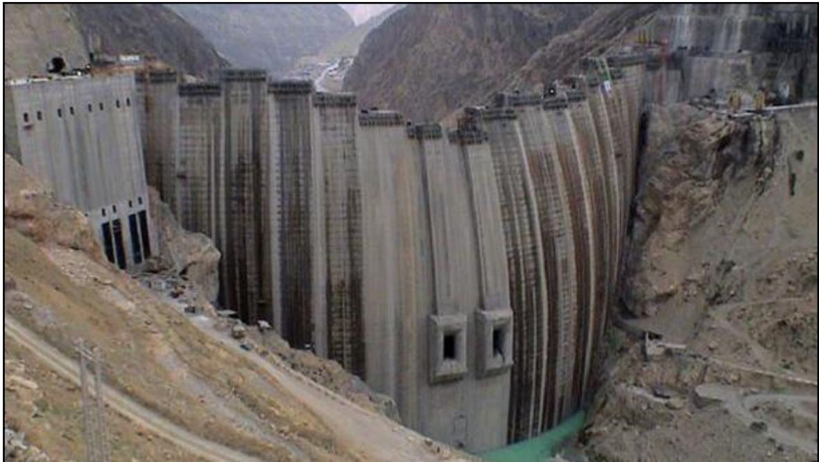
Figure 1. Construction progress at the start of Karun 4 reservoir impounding (March 25, 2010)
