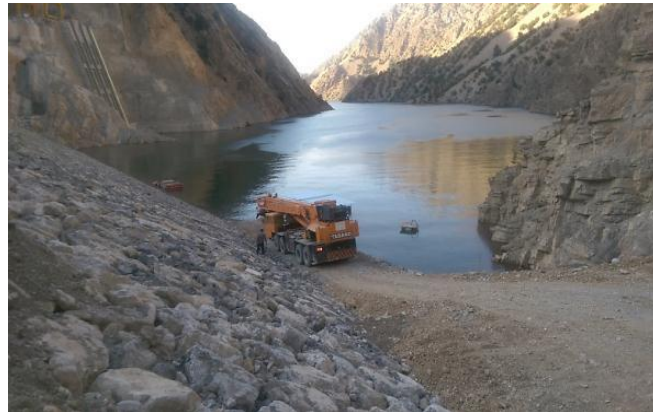
Figure 4. Location of crane
