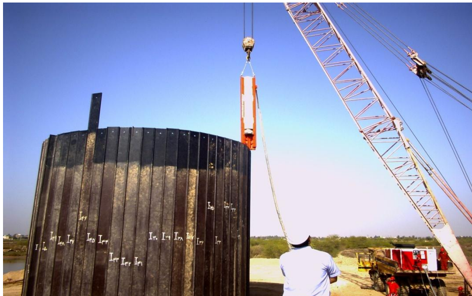
Figure 3. Construction of Bahmanshir upstream cellular dam in Khoozestan
