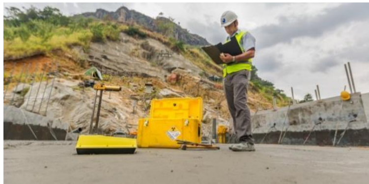
Figure 7. Density test of RCC layer by Nuclear Density Gauge
