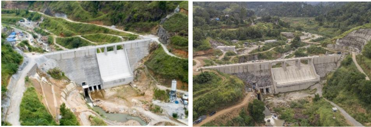
Figure 1. Downstream view of Dyraaba and Puhulpola RCC Dam
