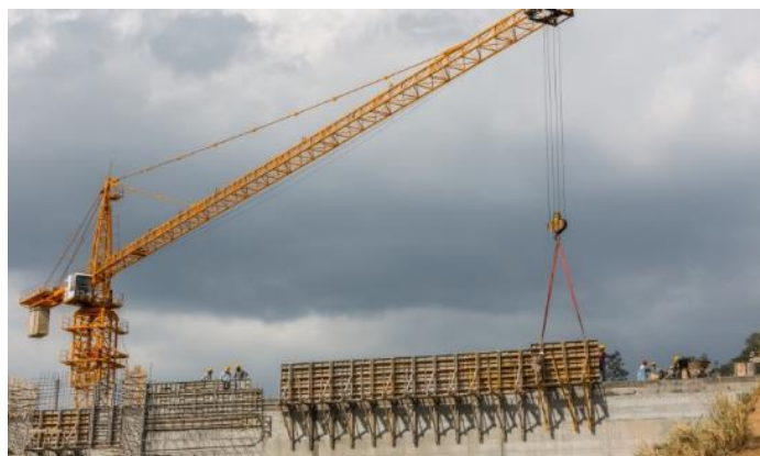
Figure 9. Forming of upstream face at Dyraaba Dam
