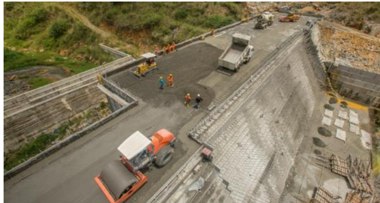
Figure 6. Transportation, Spreading and compaction of RCC
