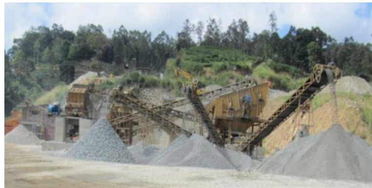
Figure 2. Aggregate production in stone crusher
