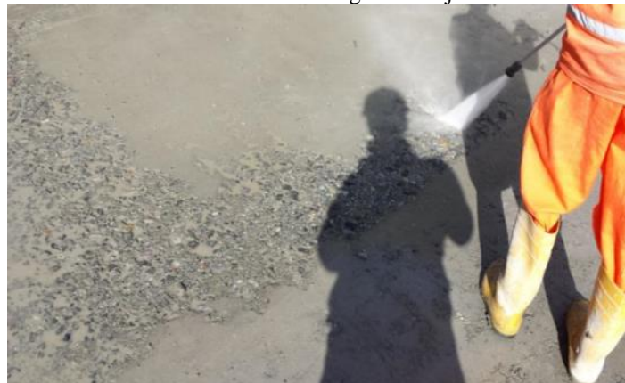
Figure 8. Green Cut of RCC surface by water jet
