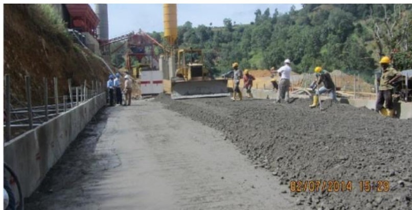
Figure 4. RCC construction of Test Pad
