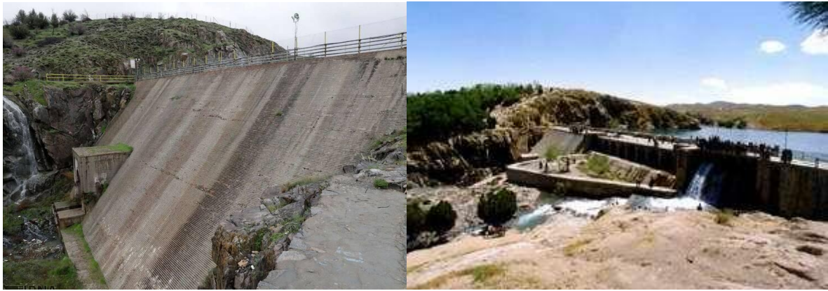
Figure 1- Downstream view of the Golestan historical dam
