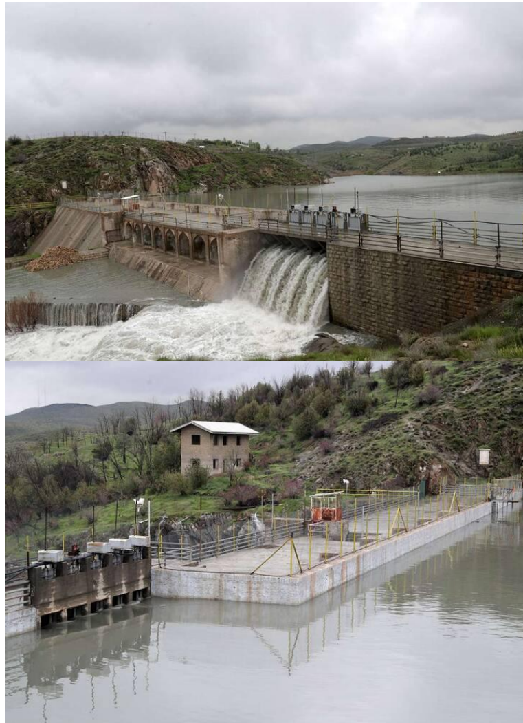
Figure 10- Acceptable performance of the retrofitted dam under 1398 flood, an environmental friendly retrofit including the upstream, downstream, crest, spillway and bottom outlet
