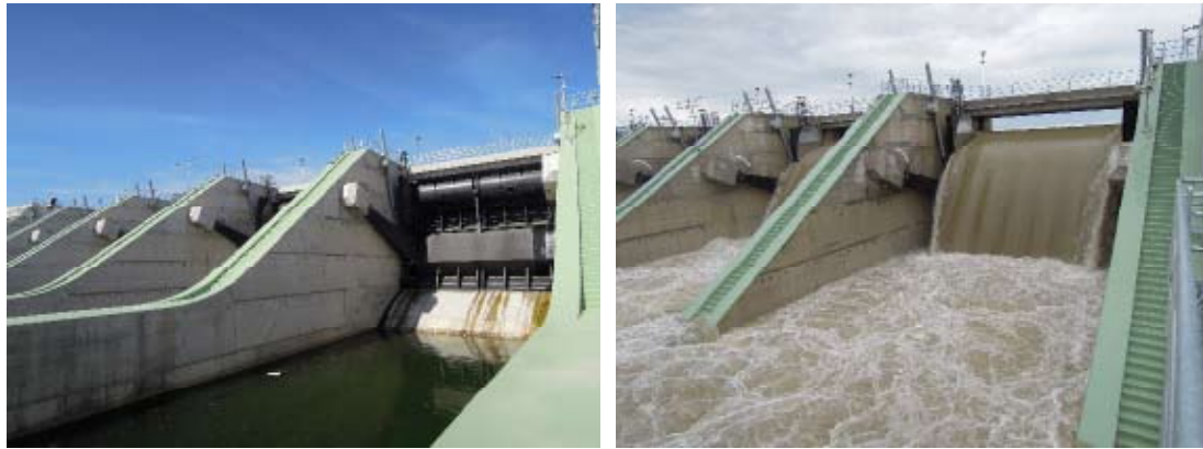
Figure 5 : Situation at Brežice dam during normal operational regime and during flood discharge.
