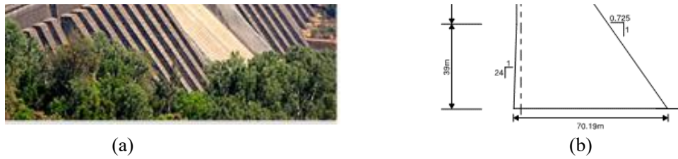
Figure 1. Koyna Dam: a) Picture of Koyna Dam b) Typical NOF monolith section.
