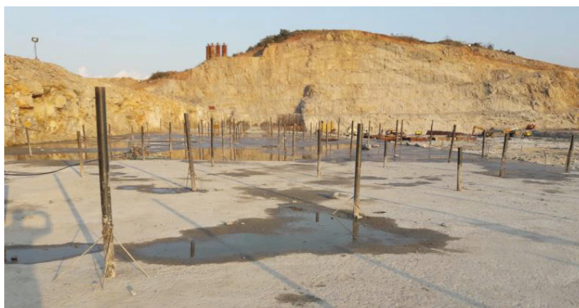
Fig. 2 : Mass concreting in progress at Polavaram Dam
