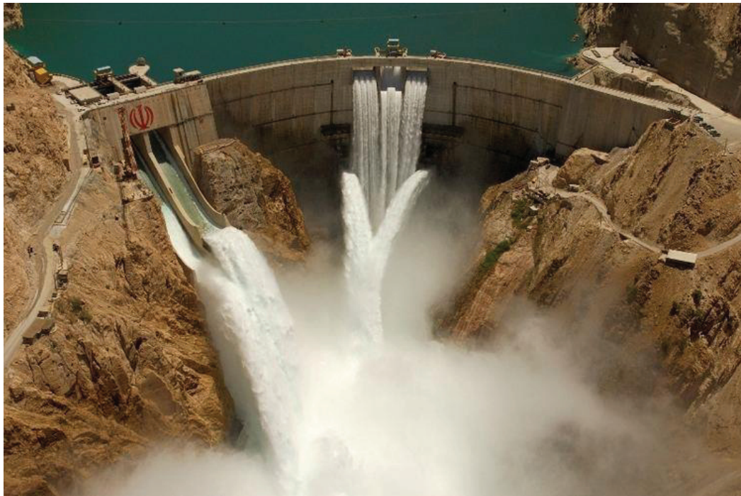
Figure 1 : Karun 3 Dam and Reservoir
