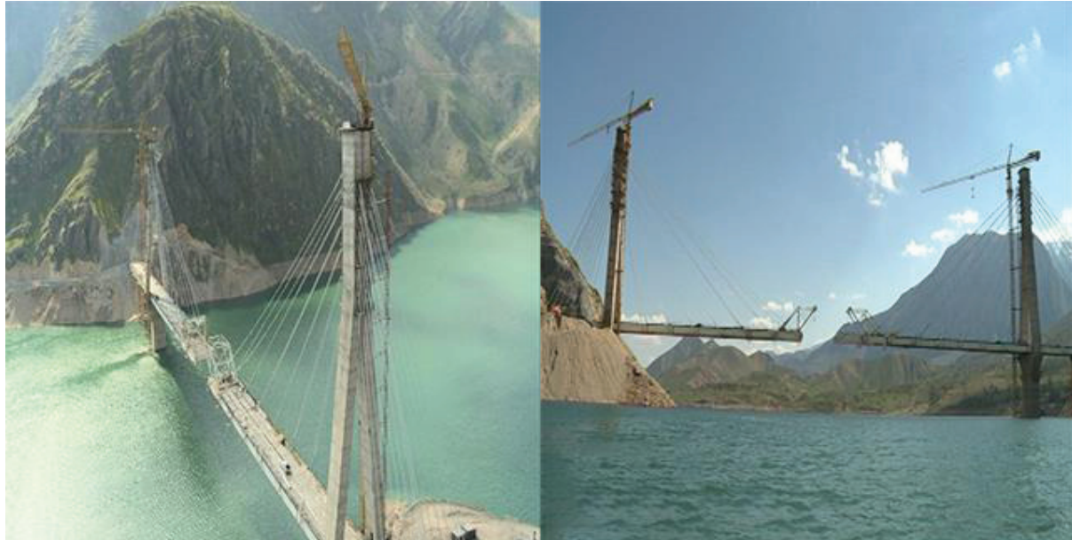
Figure 2 : Sebalutak Cable Bridge in the Karun 3 Dam Reservoir
