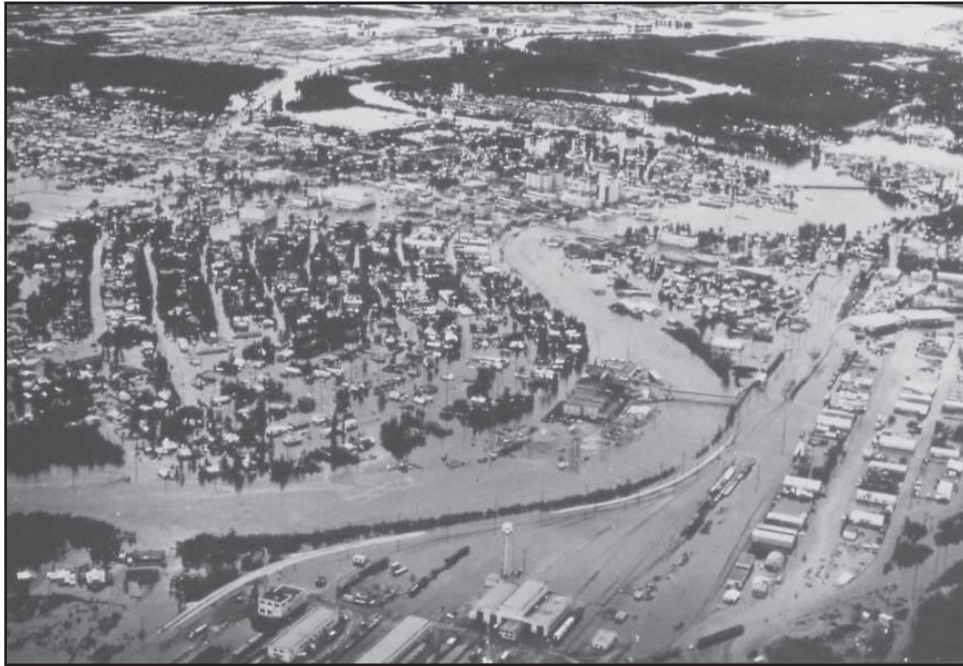
Figure 2 : 1967 flood in Fairbanks, Alaska.
