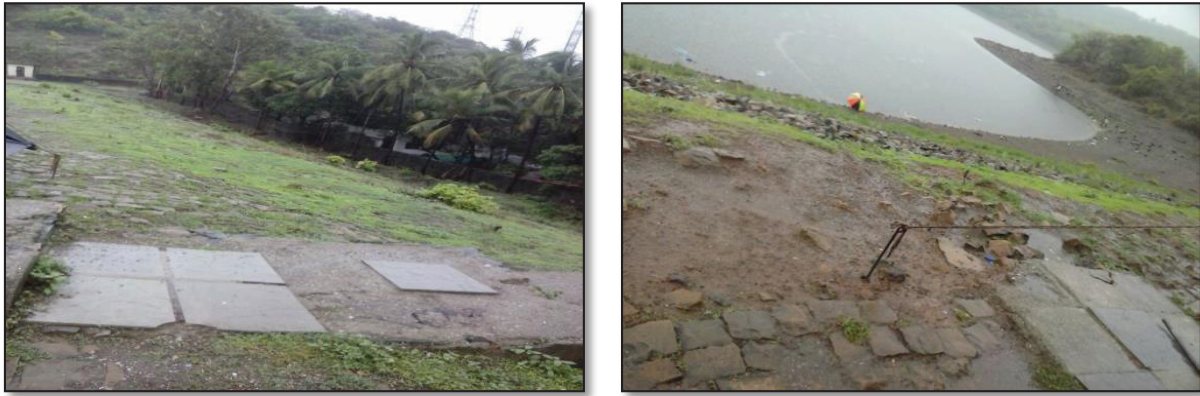
Figure 13 : Locations of Geophones at the downstream and upstream faces of the Vihar dam near Durgah
