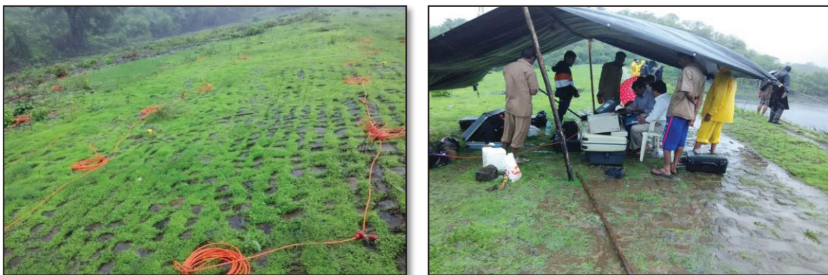
Figure 15 : Locations of Geophones at the downstream face, upstream face of the Vihar dam near Durgah
