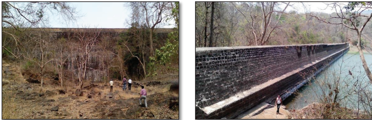
Figure 5 : Locations of Geophones at the downstream face and upstream face of the Tulsi dam No.1
