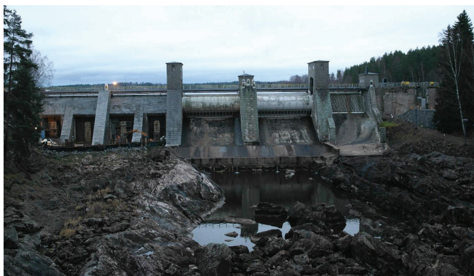
Figure 5 : Flood gates of the Imatrankoski dam. Repair works 11.12.2015.
