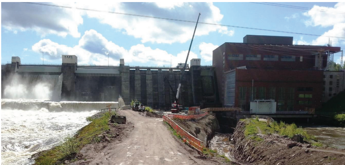
Figure 3 : Harjavalta renovation works. (Twitter.com/Harjavaltahydro 28.5.2015)
