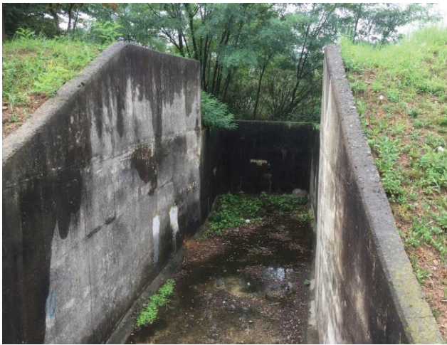
Seon-am Dam Spillway
