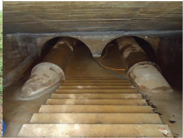
Seon-am Dam Waterway tunnel
