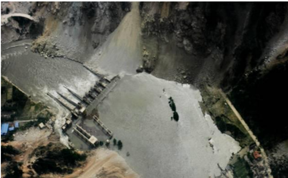
Figure 3. Overtopping of Taipingyi run-of-river power plant after the 2008 Wenchuan earthquake in China
