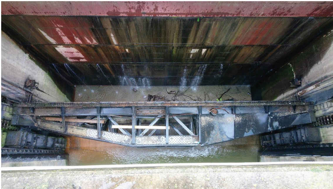
Figure 9 : The first phase of rehabilitation works - auxiliary spillway gates inserted.
