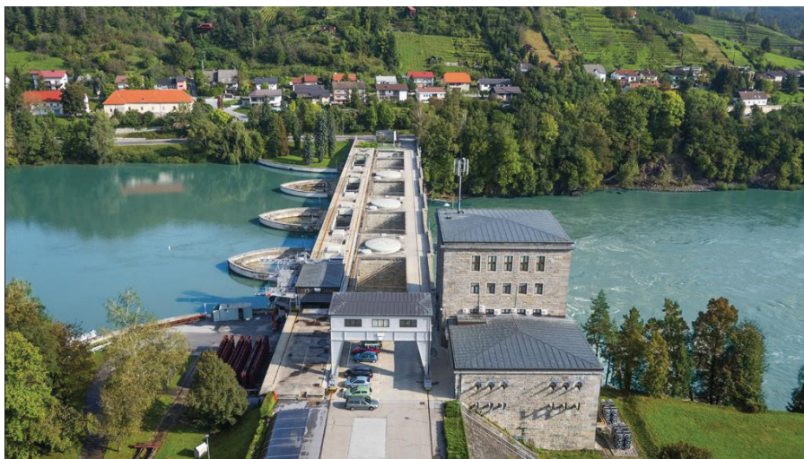
Figure 3 : Bird's-eye view of the Mariborski otok Dam.
