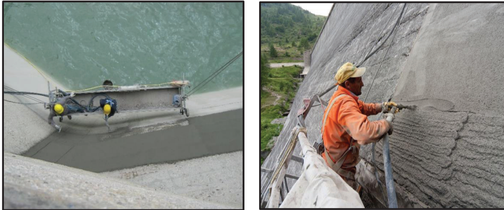
Figure 9 : Typical examples of repair with a screw pump
