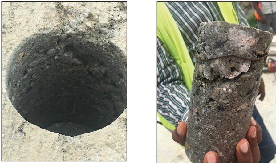
Figure 12 : Coring of a cracked concrete portion
