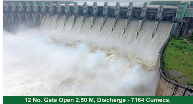
Figure 14 : Gated operation of main spillway with GO 2.5 m (Project site)
