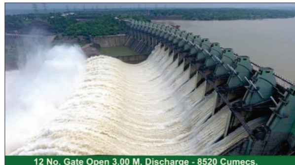
Figure 16 : Gated operation of main spillway with GO 3 m (Project site)
