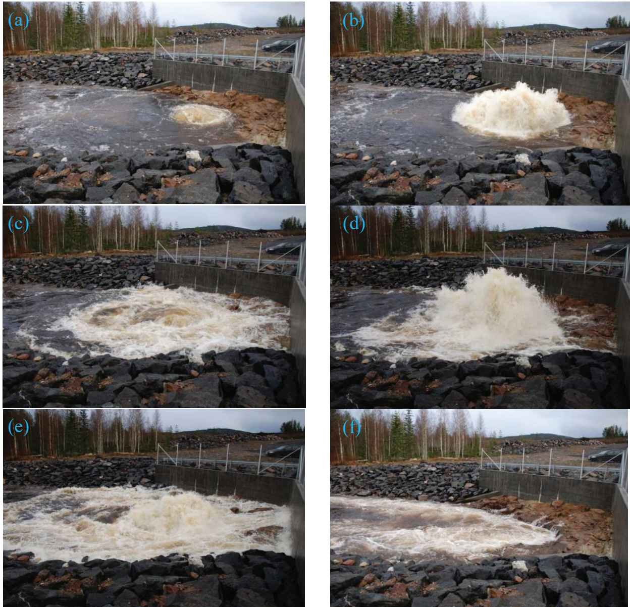
Figure 4 : Sequential blowouts at the exit, occurring at relatively small gate openings, 0.30–0.50 m.
