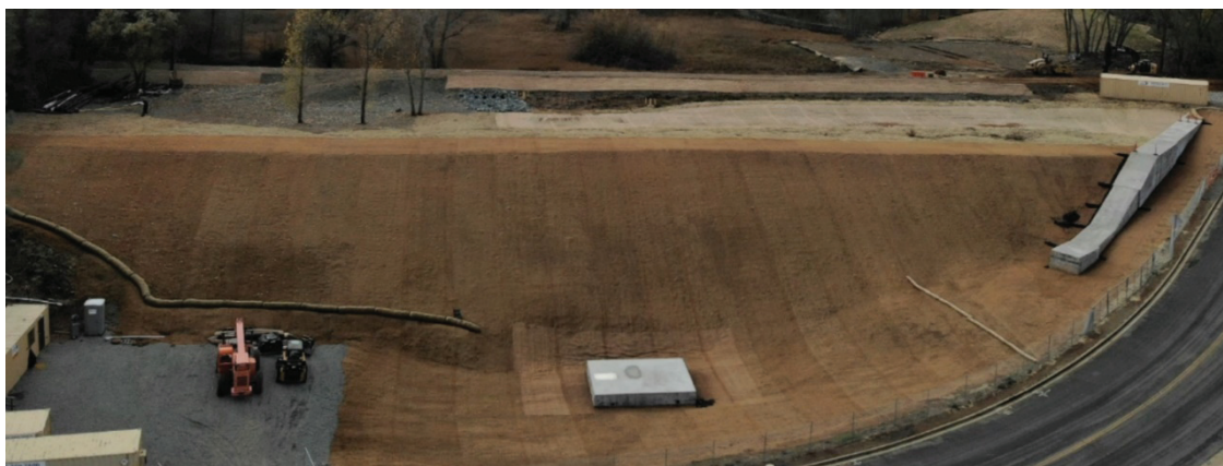
Figure 6 : Site Photo (Post Construction)
