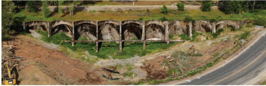
Figure 4 : Site Photo (Pre Construction)
