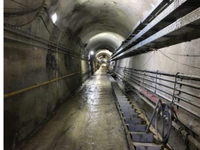
Figure 11 : Grouting Gallery with Updated Infrastructure
