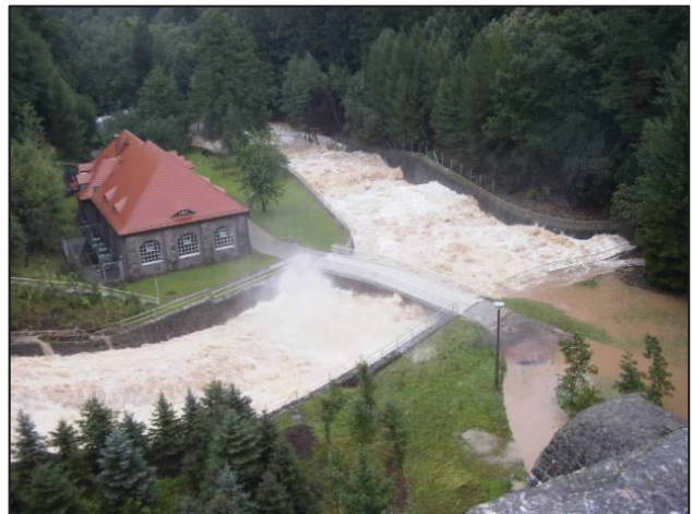
Figure 4 : Stilling basin during flood 2002 (LTV)
