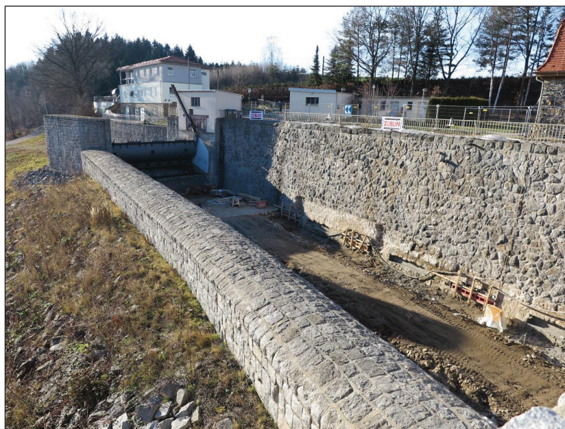
Figure 12 : Side channel – Excavation works for bottom deepening (state 12/2019)
