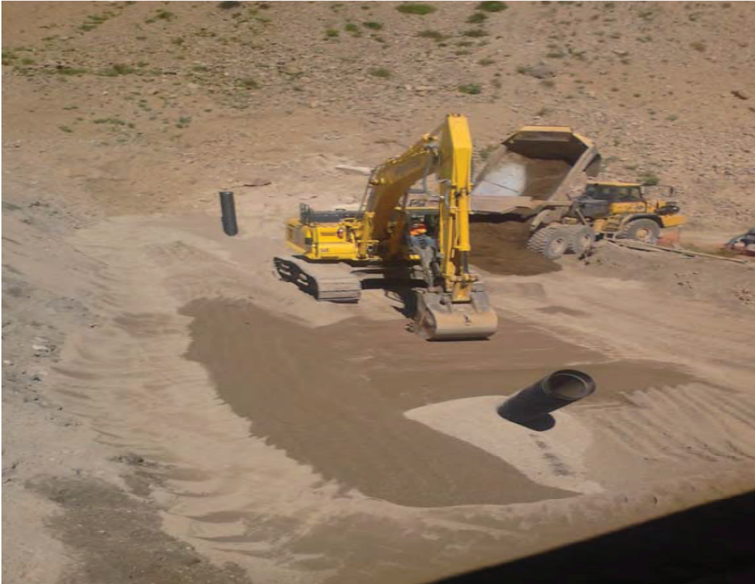
Figure 7 : Toe drain installation which included a 45 cm (18-in) diameter HDPE pipe.
