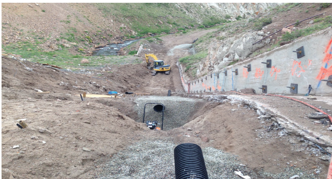
Figure 10 : Spillway chute underdrain system during construction.
