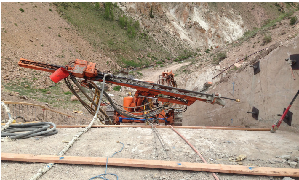
Figure 11 : Chute wall anchors being installed.
