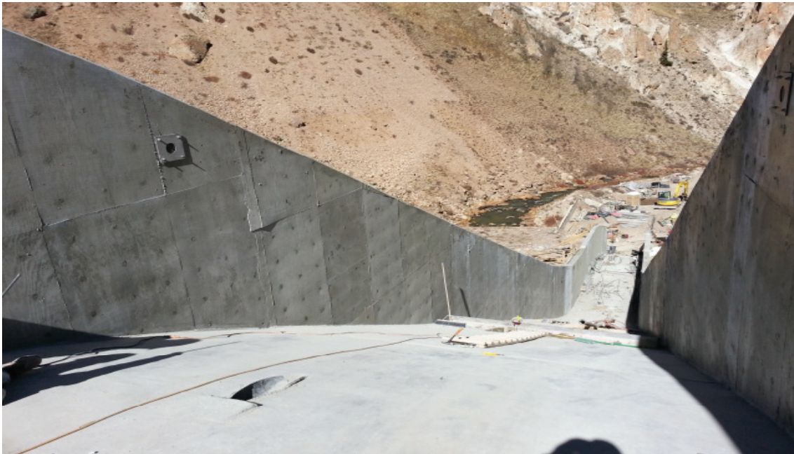
Figure 13 : Completed spillway chute walls looking downstream into the unfinished stilling basin.
