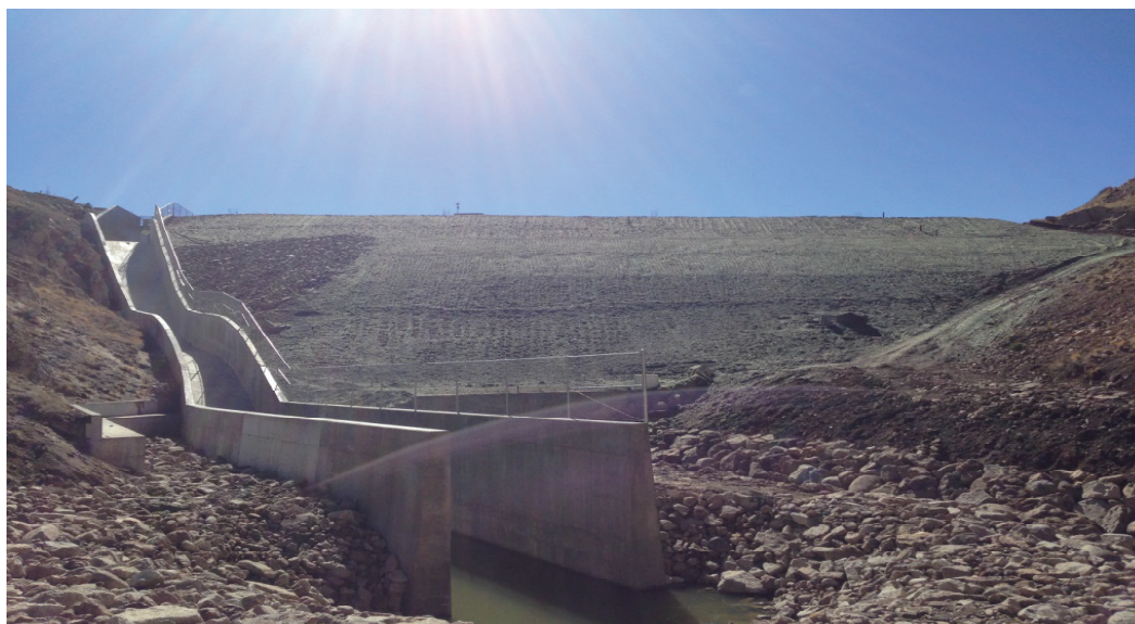
Figure 15 : View looking upstream at the completed spillway and the stability berm.
