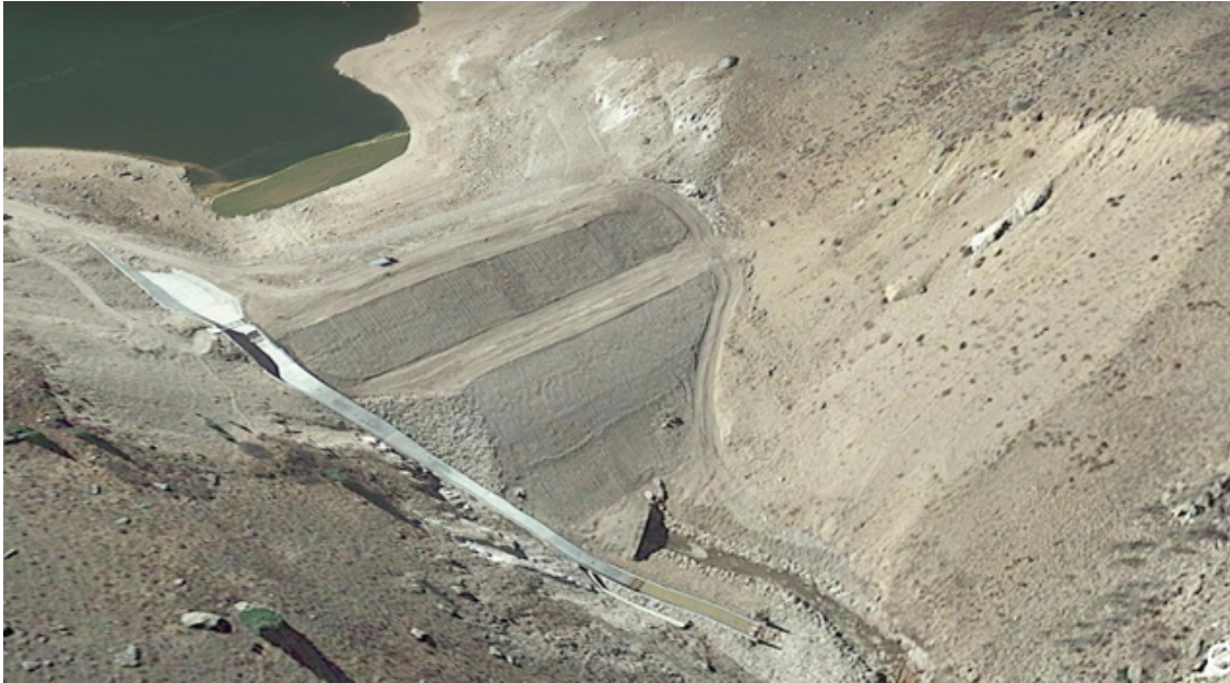
Figure 1 : Continental Dam, Colorado, USA, showing the left abutment slide area that directly contributed to mid-height, downstream dam face, seepage which was a failure mode concern.
