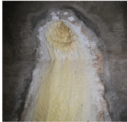
Fig. 2 : Drains are choked with calcinations
