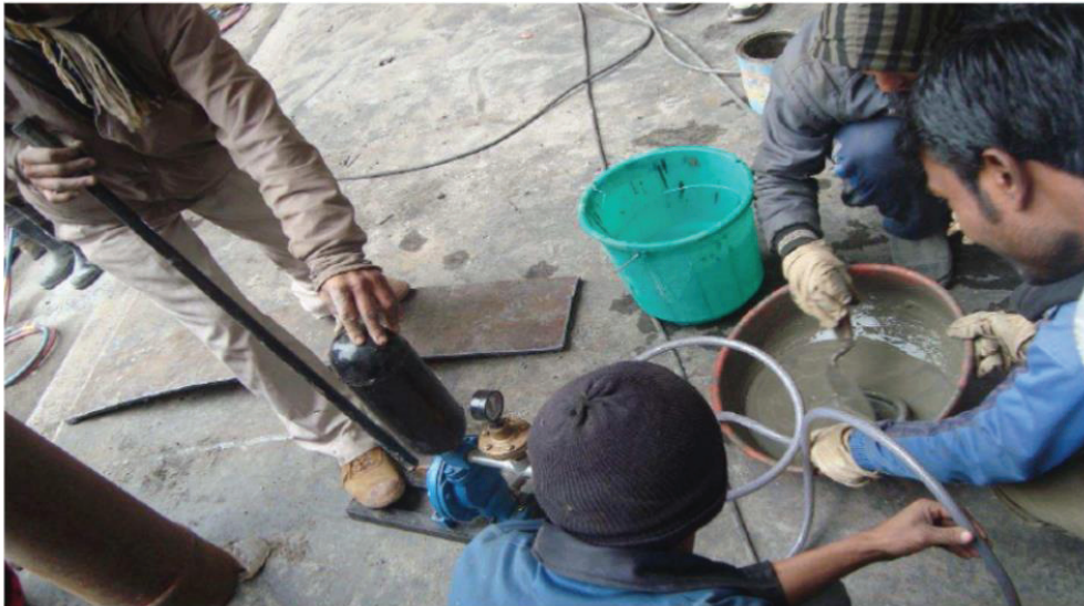
Photograph 5 : (Laying and Grouting of MS Plate in Spillway bay no 2)
