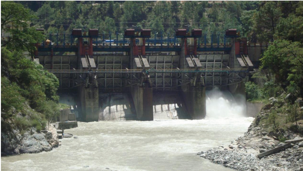
Photograph 1 : Downstream view of Maneri Dam
