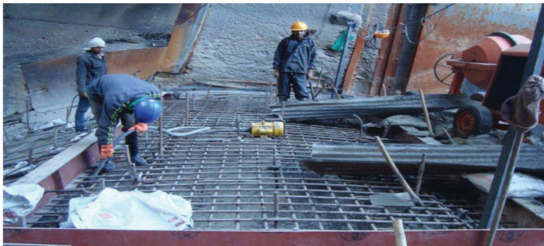
Photograph 4 : (Laying concrete in spillway bay no 2)
