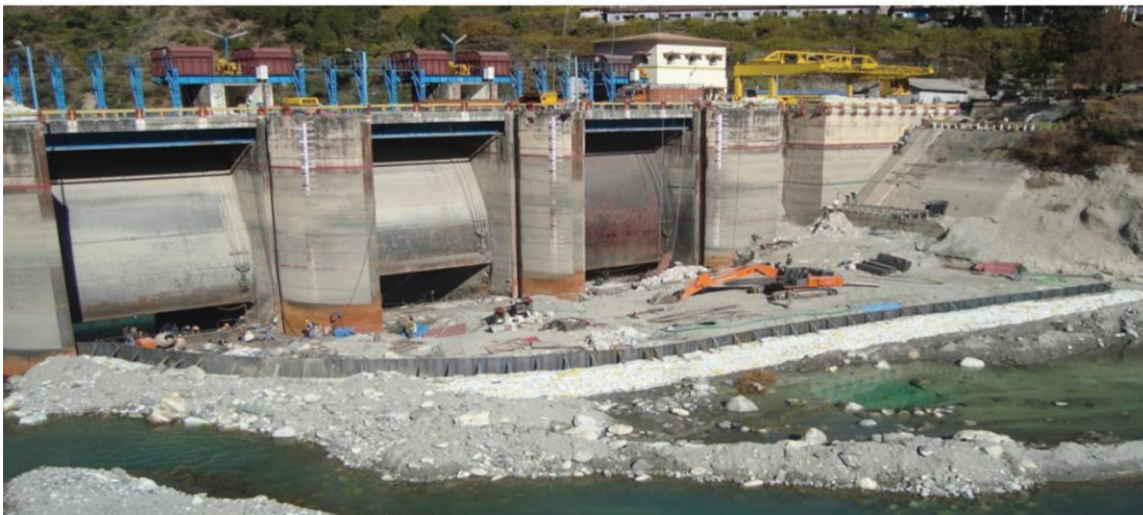
Photograph 3 : (Temporary Bund for channelization of stream water)
