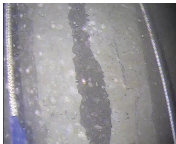
(b) After repair
