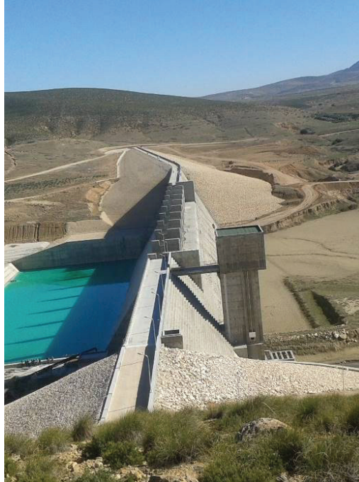
Figure 1 : Right View of Sarrath dam after construction completion (Source : N. Dhiab)
