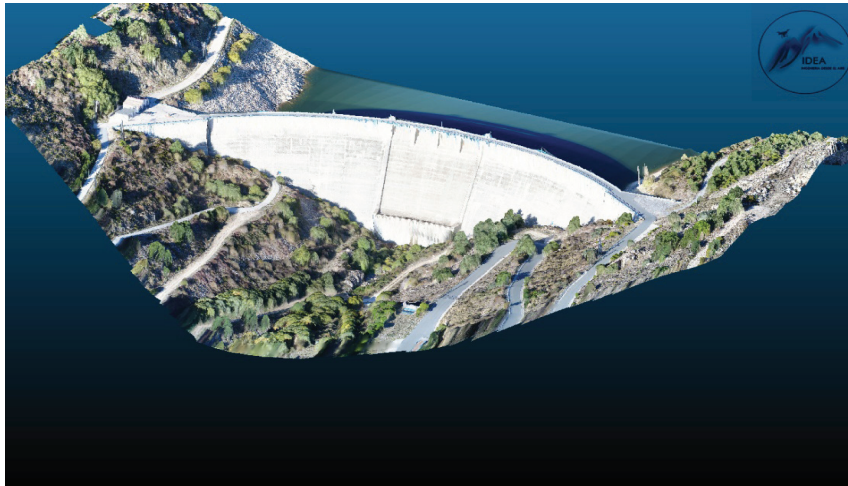
Figure 2 : 3D model with drone in a arc-gravity dam.
