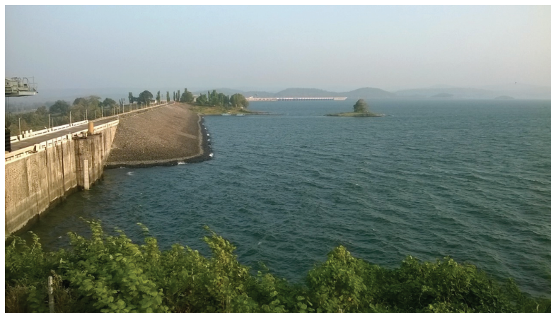
Figure 1 : Ukai Dam at upstream
