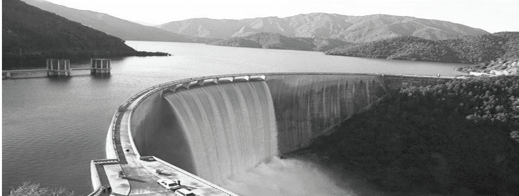
Figure 7 : Susqueda Dam overview.
