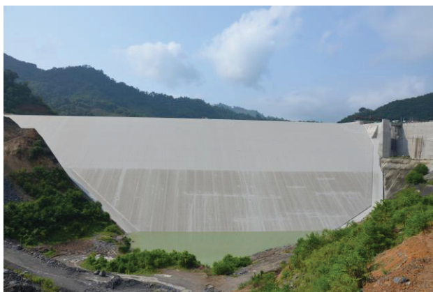
Figure5 Uncovered Composite Geomembrane Face Rock-fill Dam
