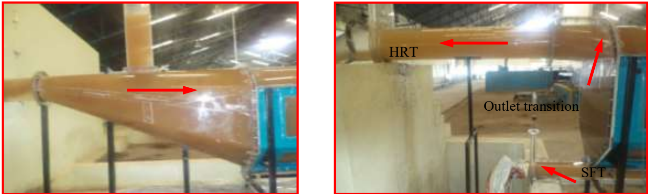
Photo 3 and 4 : View of inlet and outlet transition
