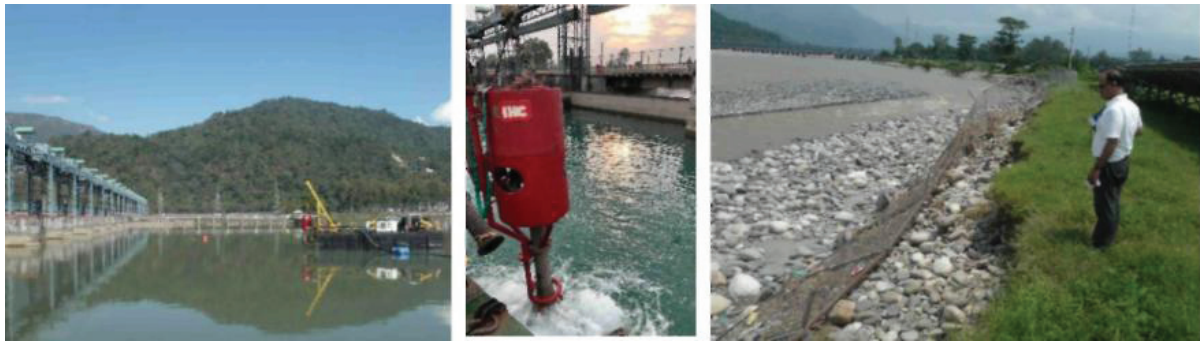
Figure 9 : The sediment handling. The left image shows the pontoon on the reservoir, the middle image shows the pump used to suck the slurry; while the right image illustrates the downstream left bank erosion and fence destruction occurred during the 2019 flood.
