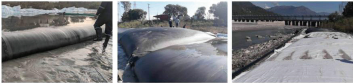
Figure 12 : Geotextile tube along the eroded bank, downstream of the barrage.
