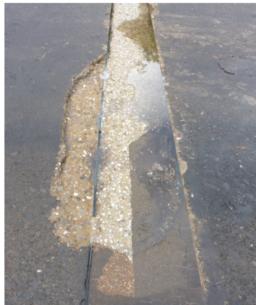
Figure 3 & Figure 4 : Damage of joints at Dam A
