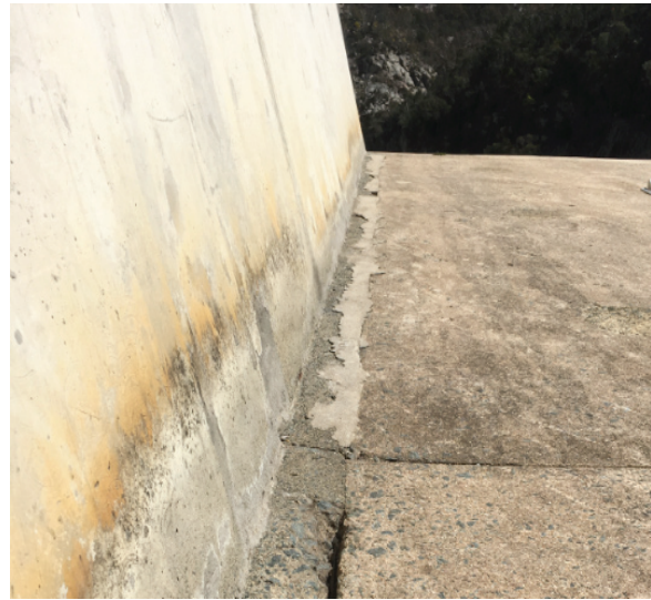
Figure 6 and Figure 7 : Damage of points of wall interface
