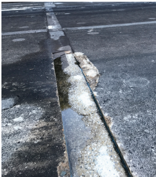
Figure 3 & Figure 4 : Damage of joints at Dam A
