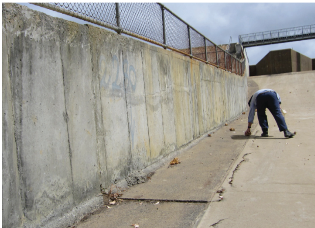
Figure 11 & Figure 12 : Damage of concrete slabs at wall interface
