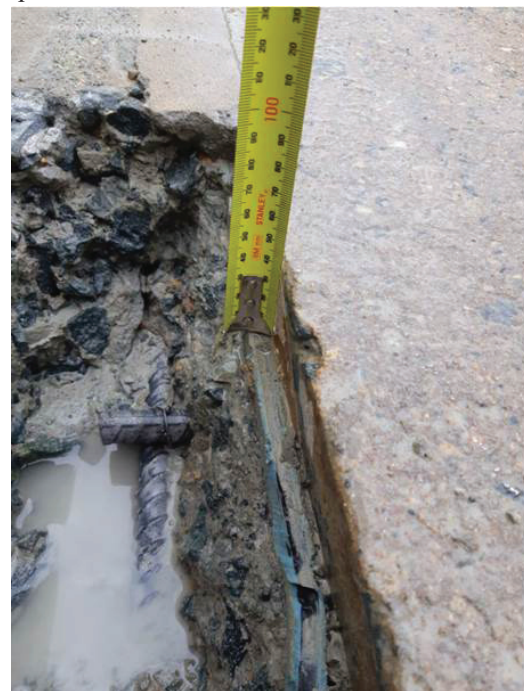
Figure 8 and Figure 9 : Exposure of waterstop at joint at Dam B
