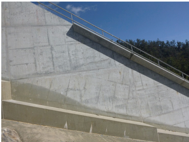
Figure 15 : Newly constructed wall
