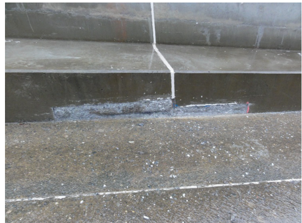
Figure 16 : Removal of damaged concrete
