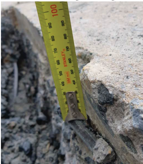
Figure 8 and Figure 9 : Exposure of waterstop at joint at Dam B
