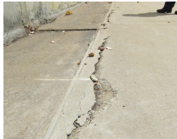
Figure 11 & Figure 12 : Damage of concrete slabs at wall interface
