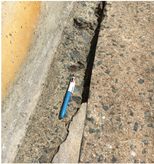
Figure 6 and Figure 7 : Damage of points of wall interface
