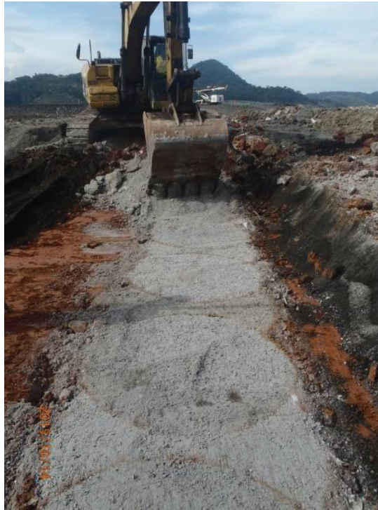
Figure 12 : Trimming the top of the cutoff secant-pile wall
