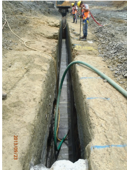
Figure 6 : Cleaning of concrete cutoff wall trench
