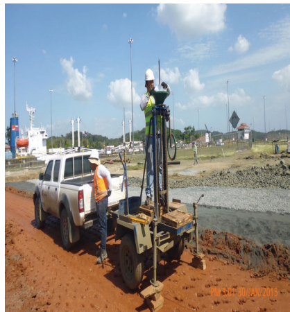
Figure 9 : Vane shear testing of compacted core material
