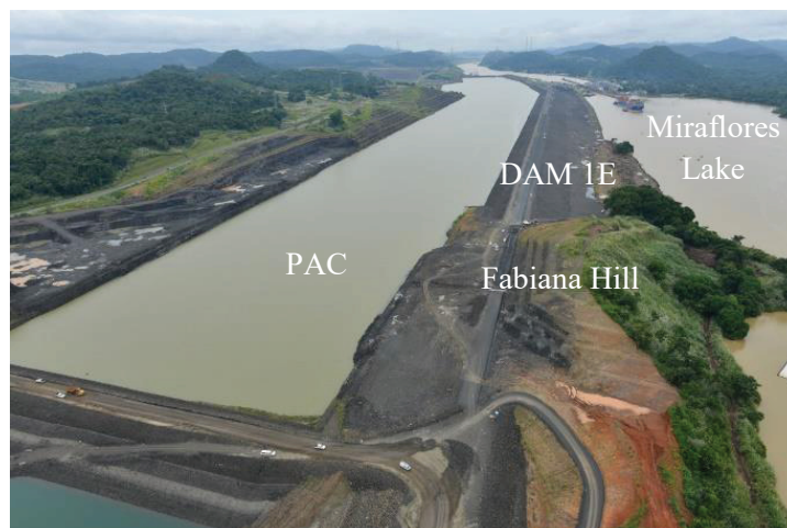
Figure 1 : View of Pacific Access Channel (PAC) and Dam 1E, looking North
