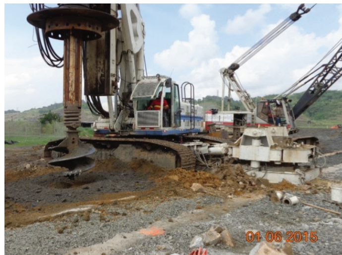
Figure 11 : Excavation of secant piles
