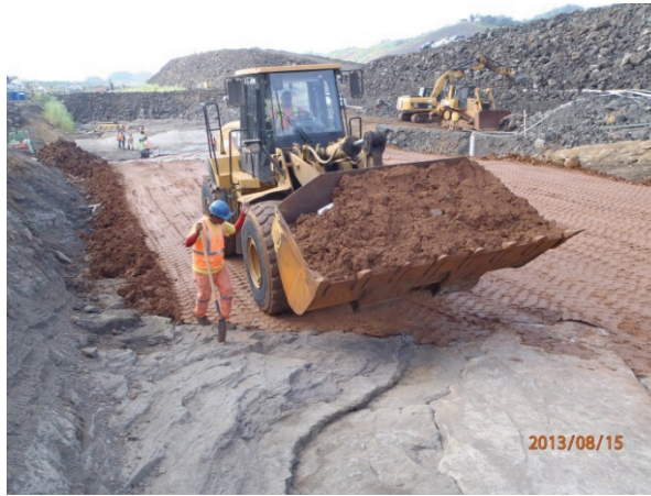
Figure 8 : Compaction of core Zone 1A with front-end loader
