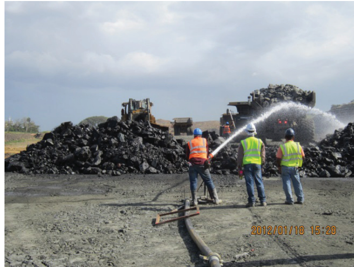
Figure 10 : End-dumping, spreading, and watering of shoulder rockfill
