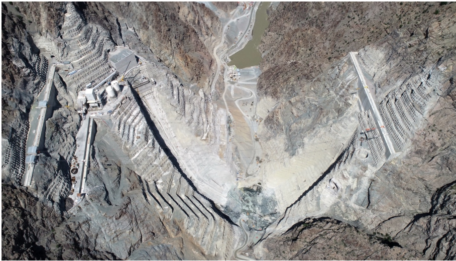
Figure 2. Yusufeli Dam site on completion of excavation
