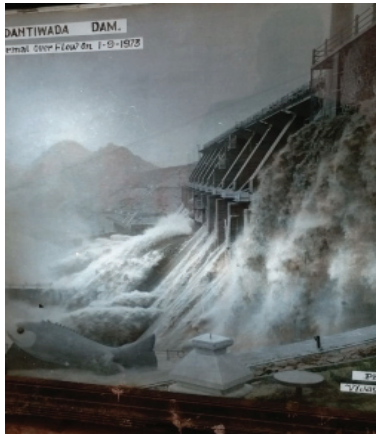
Figure 7 : Dantiwada Dam – actual flood much more than the design flood
