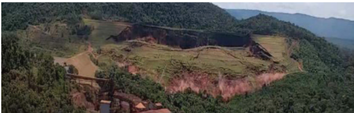
Figure 1 : Failure of the Feijão Dam (Robertson et al, 2019)
