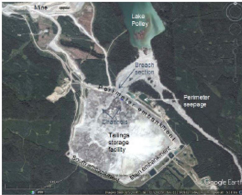
Figure 6 : Satellite image of the Mount Polley tailings storage facility and the surrounding area one day after the breach occurred (Source: Google Earth)
