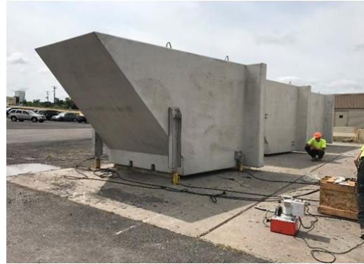
Fig. 12 Fusegate jacking to verify ballast requirements F..
