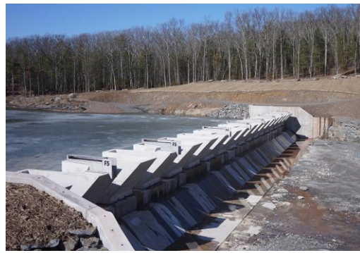
Fig. 15 Completed Fusegate System at Pikes Creek E..
