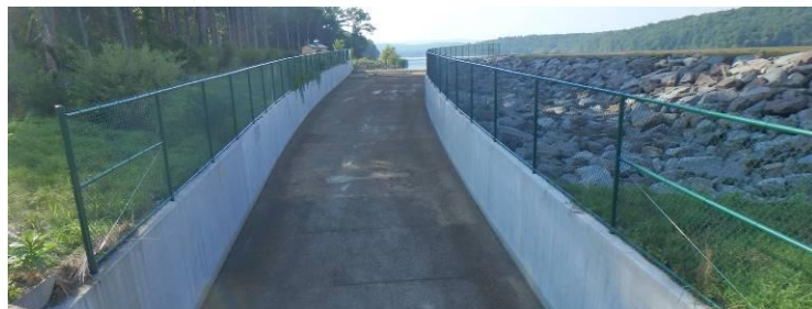
Fig. 3 Principal spillway chute and left wall berm (looking upstream) F..
