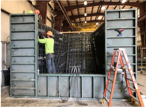
Fig. 11 Custom-made formwork and steel placement F..
