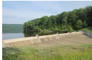
Fig. 2 View of auxiliary spillway F..
