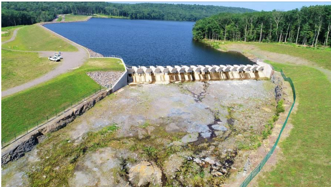
Fig. 16 Completed Auxiliary Spillway at Pikes Creek E..
