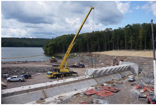
Fig. 14 Fusegate Installation at Pikes Creek E..
