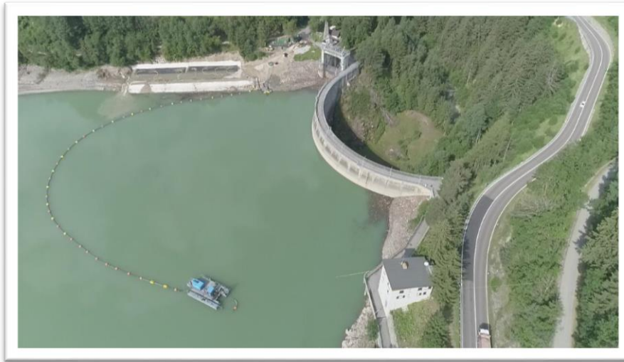
Figure 7. Aerial view of the dredging activity
