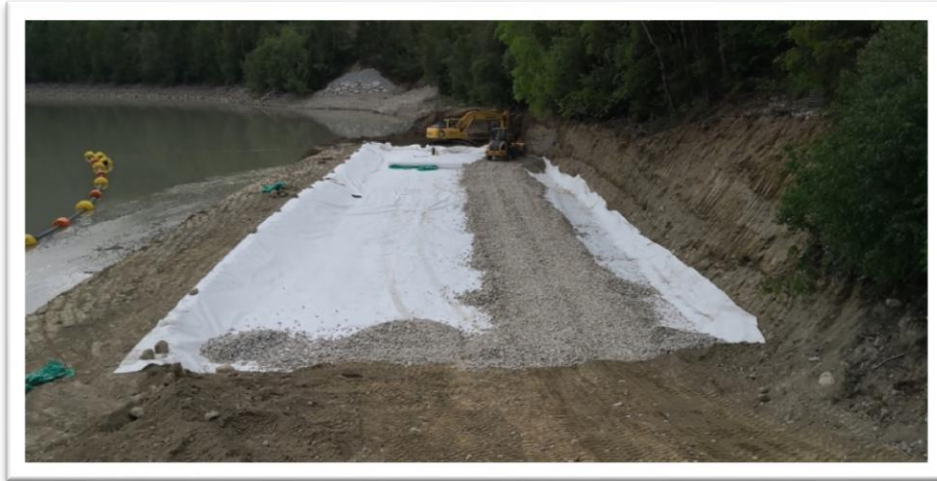
Figure 9. Final disposal area preparation (granular material over the geotextile)
