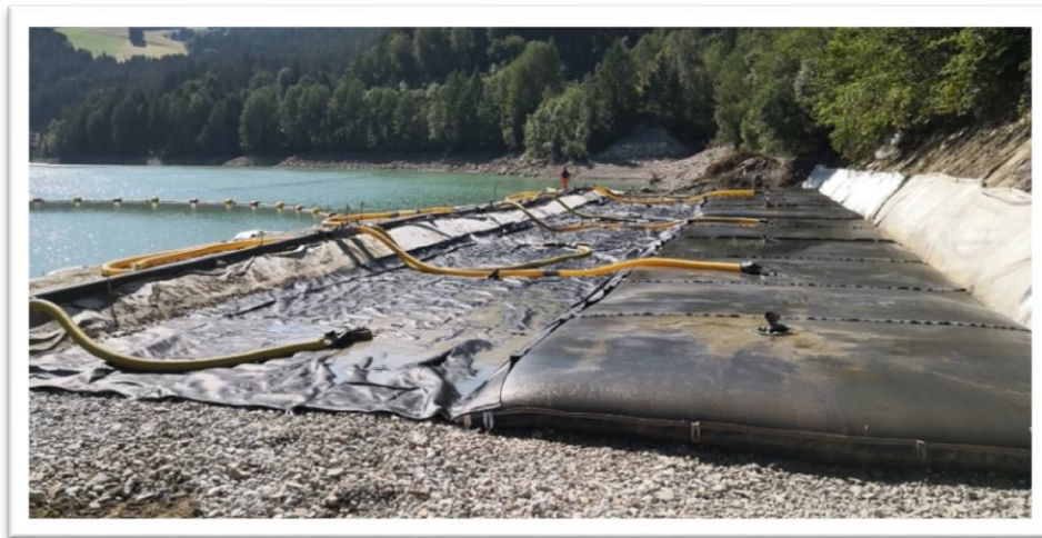
Figure 10. Geotextile tube filling
