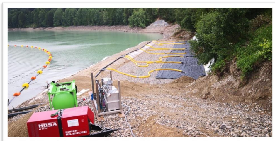
Figure 11. Flocculant mixing plant
