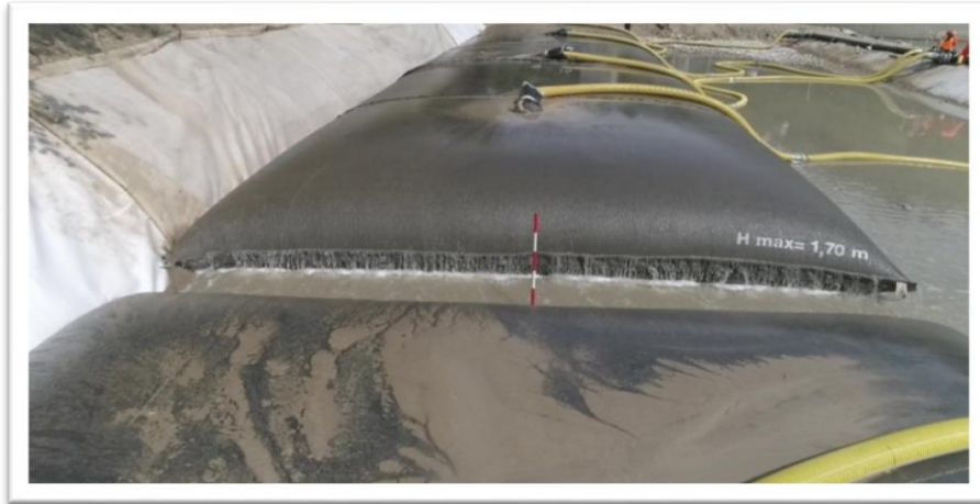
Figure 12. Dewatering of dredged sediments
