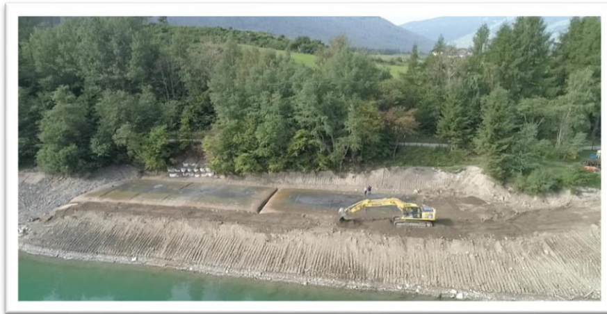
Figure 13. Final covering of the geotextile tubes with soil
