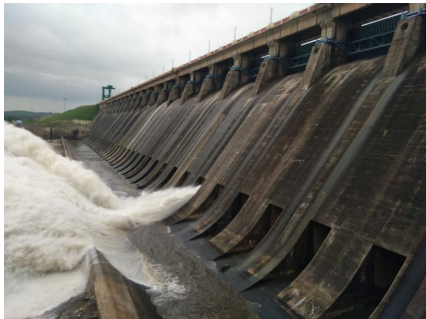
Fig.2: View of LHS Spillway along with Under Sluices
