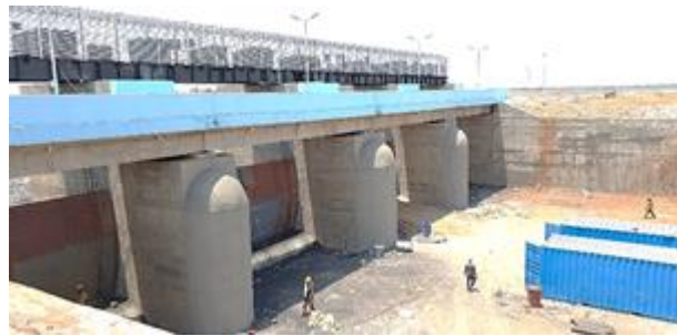
Figure 6. Manimukthanadi dam additional spillway
