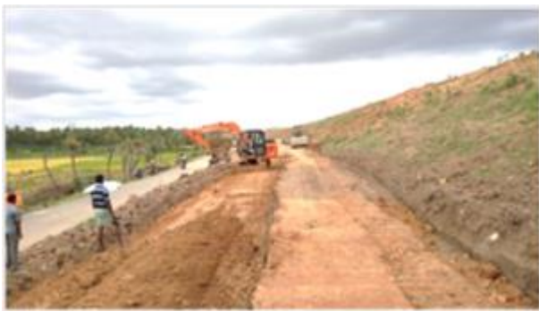
Figure 12. Mallaghata dam re-sectioning.
