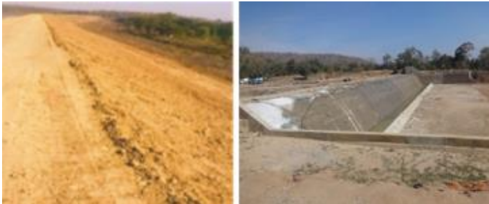
Figure 7. Sarathi dam raised and weir modified to ogee.
