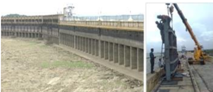
Figure 9. Replacement of 136 gates at KRS dam.
