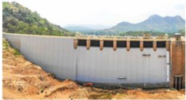
Figure 15. Servalar dam geomembrane treatment
