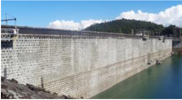
Figure 14. Porthimund dam u/s face treatment.
