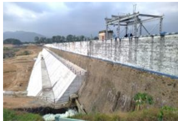
Figure 11. Pechiparai dam backing concrete.
